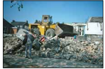
Demolition work underway at Tow Law
